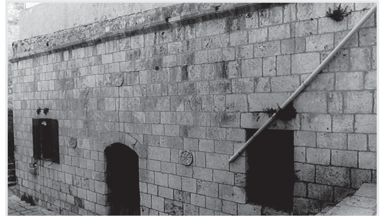
Pl.4.17 The north façade of the Kitchen of al-Imara al-Amira
