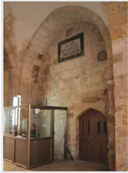
Pl.4.11 The east wall of the south entrance vestibule
