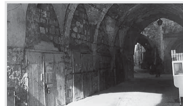
Pl. 3.4 Eastern elevation of Ribat Bairam Jawish (before)
