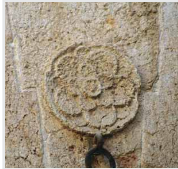
Pl.4.7 Decorative roundel at the middle of the north door lintel
