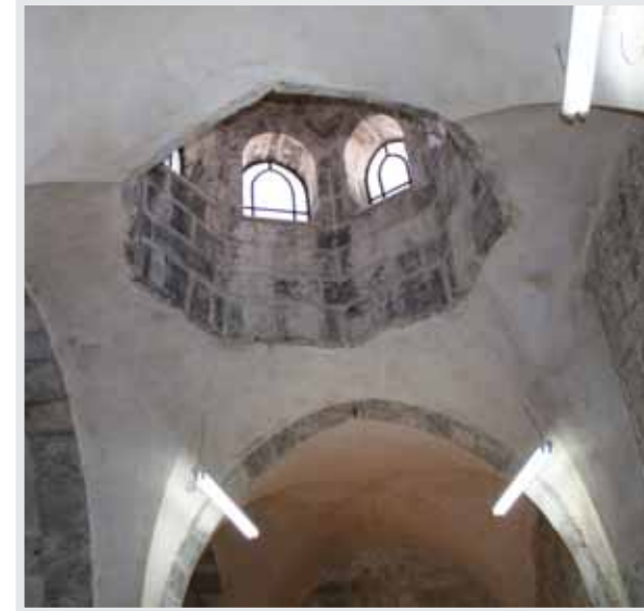
Pl.4.19 The dome of al-Imara al-Amira Kitchen (from interior)
