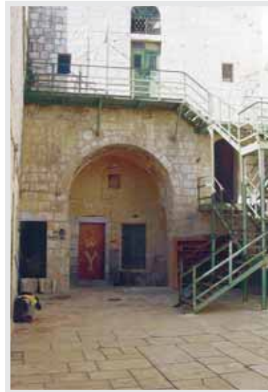
Pl.1.12 End of the stairs of western entrance of Dar al-Sit Tunshuq al-Muzafariyya
