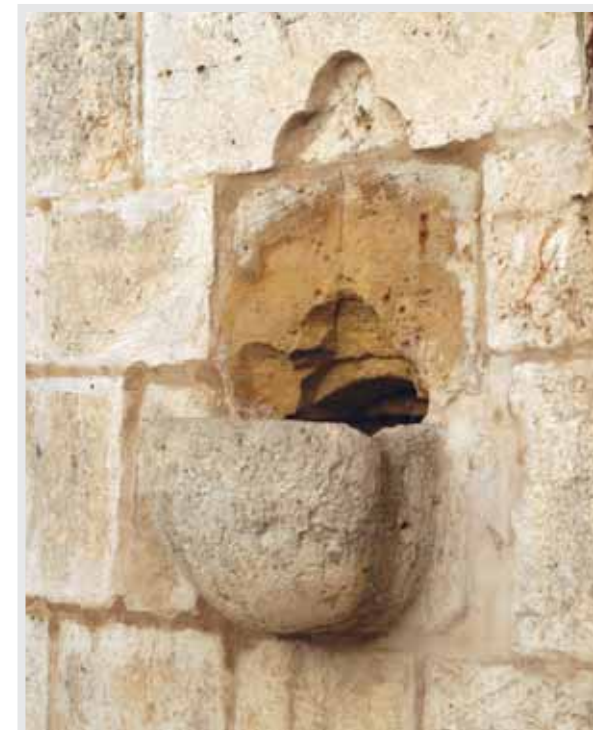
Pl.4.18 Water basin of façade kitchen of al-Imara al-Amira
