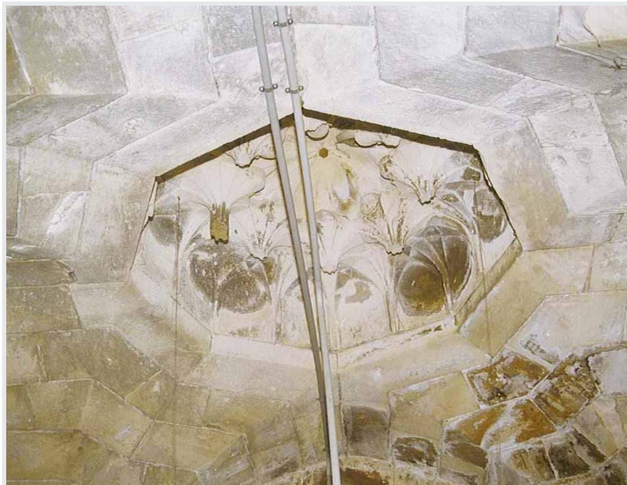
Pl.1.10 Covering of the vestibule of the eastern portal
