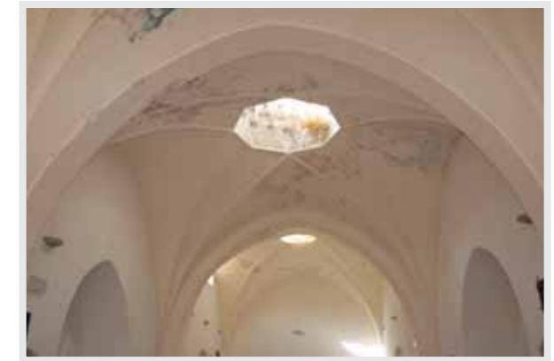
Pl.1.15 Roof covering of the durqa'a in Dar al-Sit Tunshuq al-Muzafariyya
