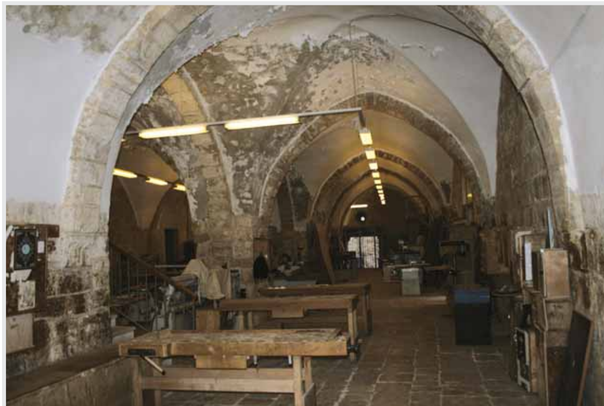
Pl.1.8 Main hall of the first floor of Dar al-Sit Tunshuq al-Muzafariyya
