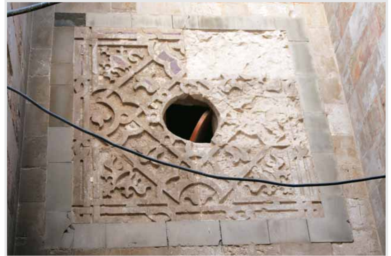
Pl.1.7 Details of the stone panel of the eastern portal of Dar al-Sit Tunshuq al-Muzafariyya
