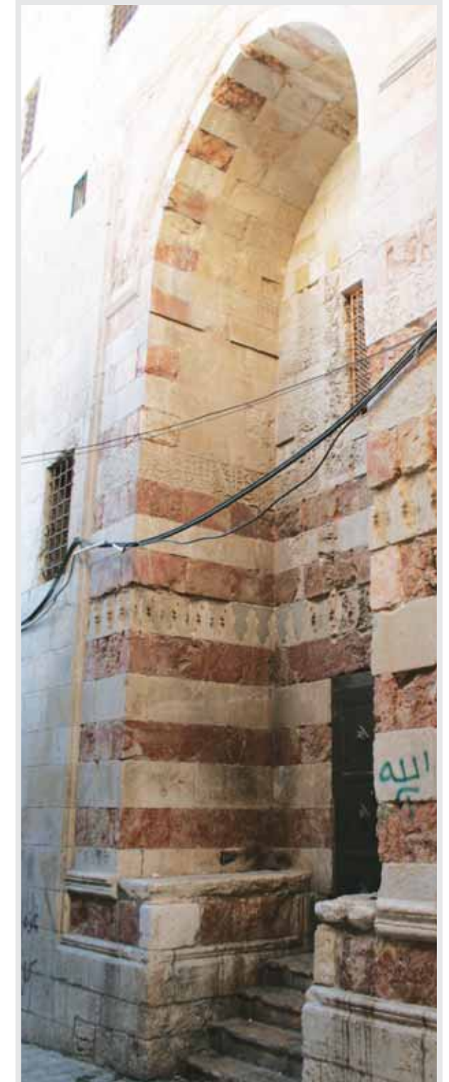
Pl.1.2 Western portal of Dar al-Sit Tunshuq al-Muzaffariyya
